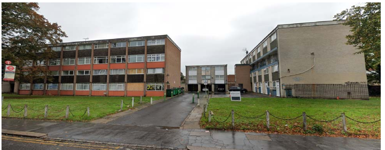
Figure 3: Existing buildings on site (viewed from Wellesley Road)
